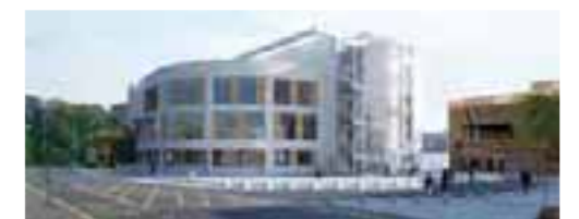
Green Street, Kilmarnock
